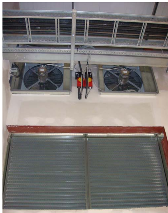
The air economiser (shown in these images) design by Capitoline helped give this Data Centre one of the best PUE in the industry,
