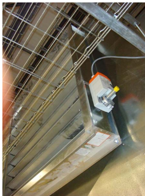
The air economiser (shown in these images) design by Capitoline helped give this Data Centre one of the best PUE in the industry,
