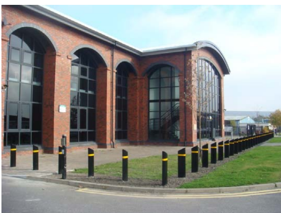
Welsh Government data centre, South Wales
