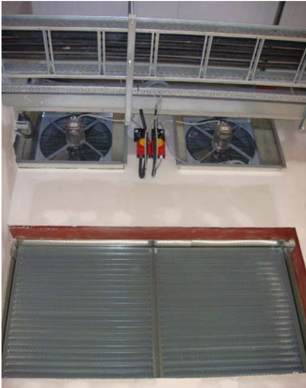
Above: Construction of the air economiser Top right: Capitoline plans for cable layout Right: The new building Below: The main computer hall
